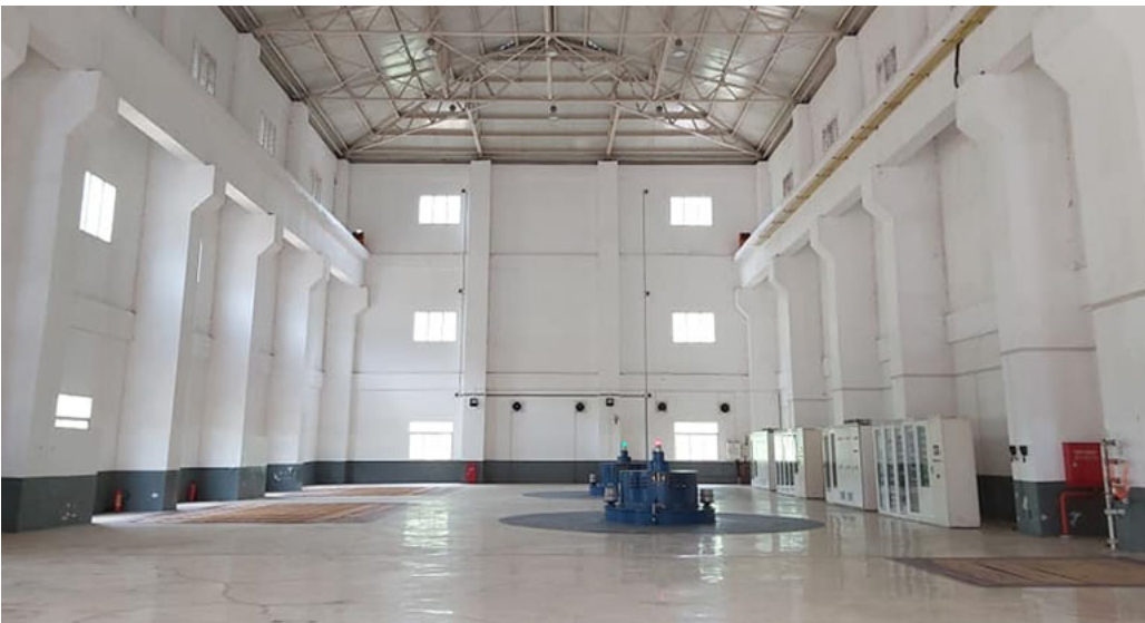
Nam Chiane 1 dam structure images shown below:
